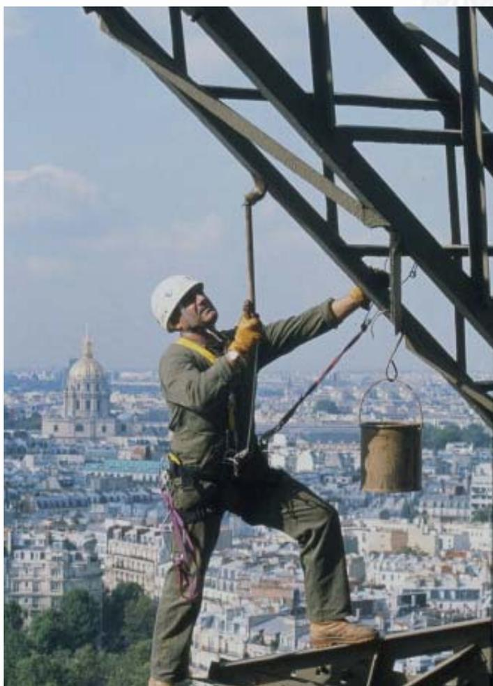
Painters painting the Tower using a roll attached to the end of a brush (long brush)
