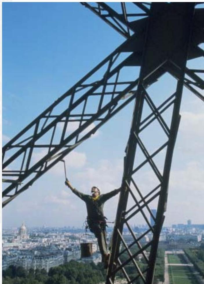
disks and 60 tons of paint. To ensure the workers' safety, 50 km of safety ropes and 2 hectares of protective nets are installed.
